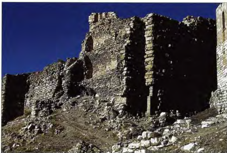
The rock-cut fosse that separated the spur-castle at Karak from the rest of the hill on the right is shallow compared to the example at Saone. This section of the outer wall dates from the late-1160s, while the structure behind is believed to date from the first Crusader castle, built around 1142.
